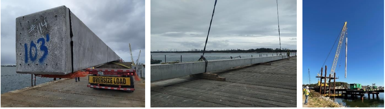
Figure A - 31. Pile delivery and handling
