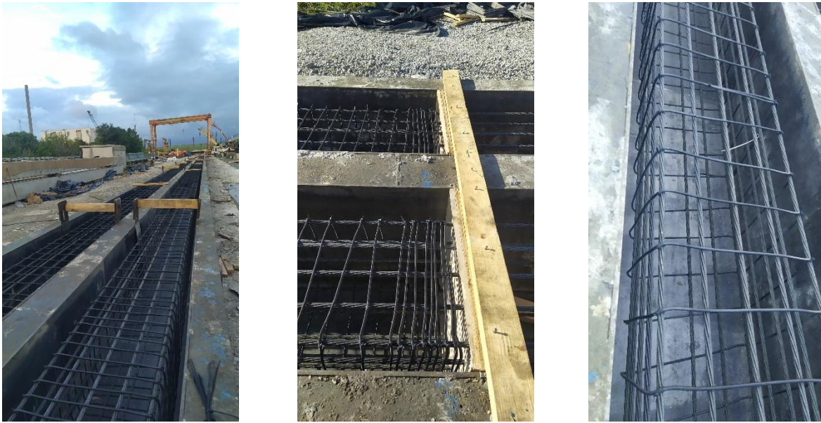
Figure A - 24. Piles at prestressing beds
