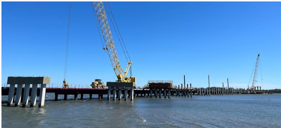
Figure A - 15. CFRP prestressed concrete piles and early pile cap construction
