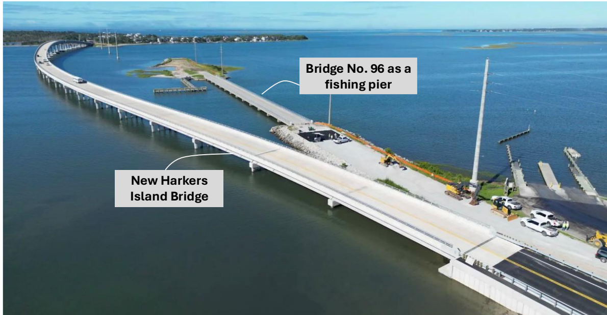
Figure A - 18. Completed Harkers Island Bridge
