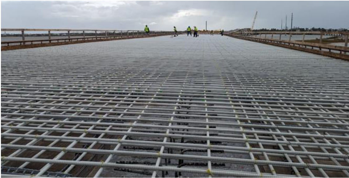
Figure A - 13. Deck GFRP reinforcement
