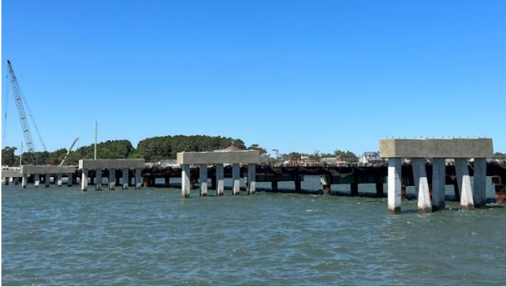
(a) Pile caps directly on piles
