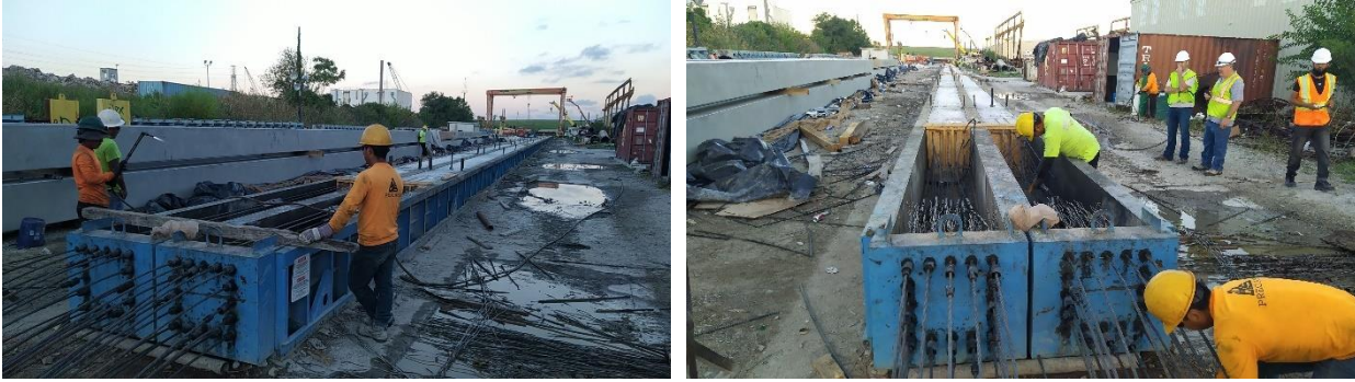
Figure A - 28. Detensioning of piles
