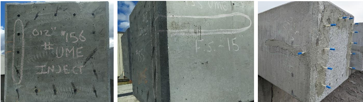
Figure A - 30. Pile crack repairs
