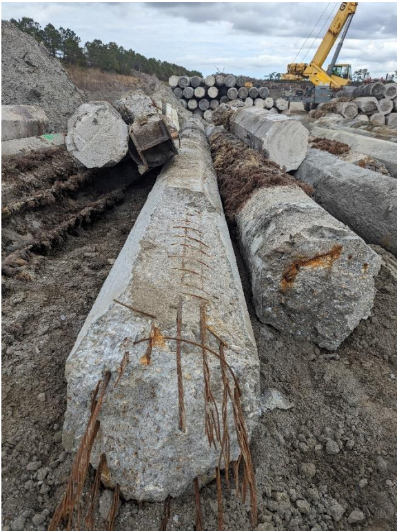
Figure A - 53. Demolished octagonal piles from Bridge No. 73
