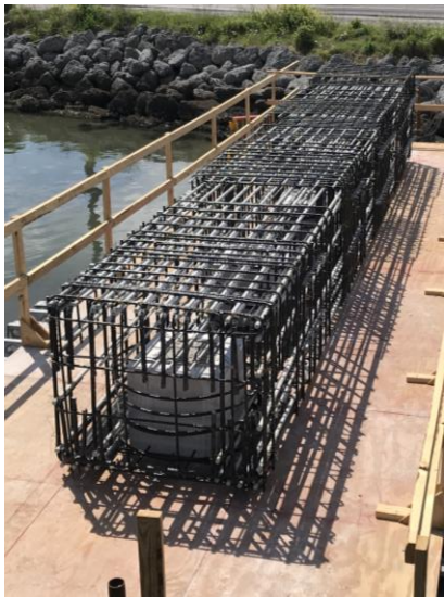
(a) Pile cap reinforcement cage
