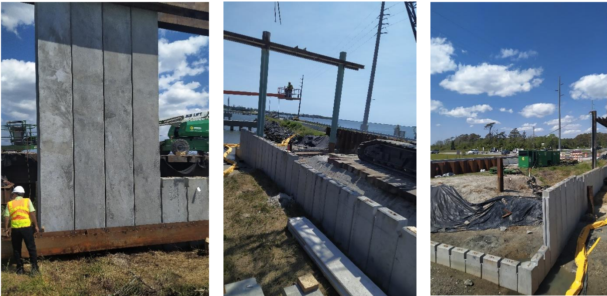
Figure A - 41. Retaining walls on the mainland side
