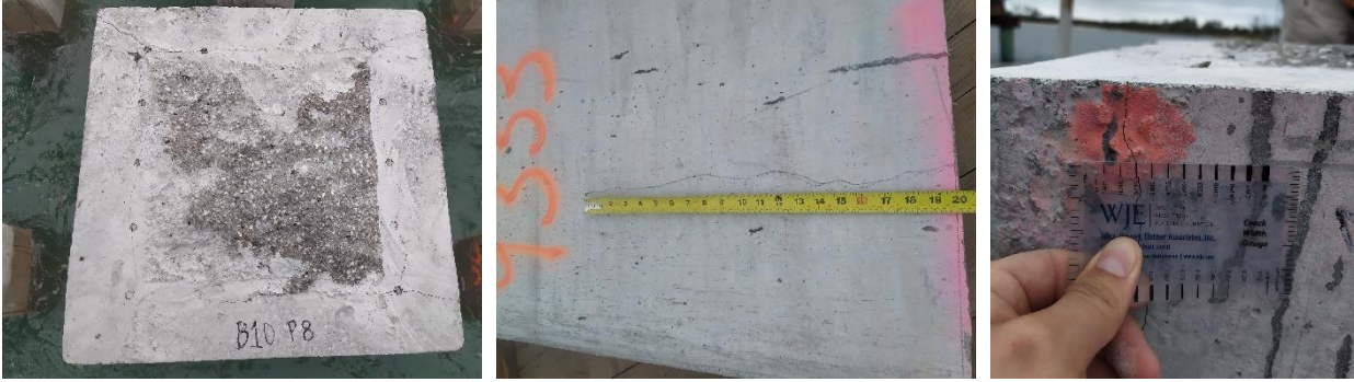
Figure A - 34. Pile cracking at cut-off ends
