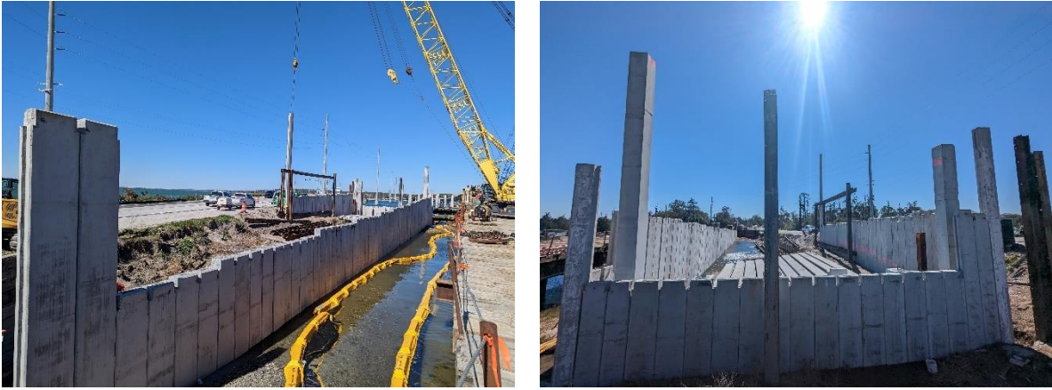
Figure A - 42. Retaining walls on the island side
