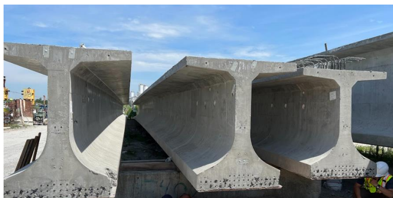
Figure A - 10. 54 in. CFRP-prestressed FIB girders
