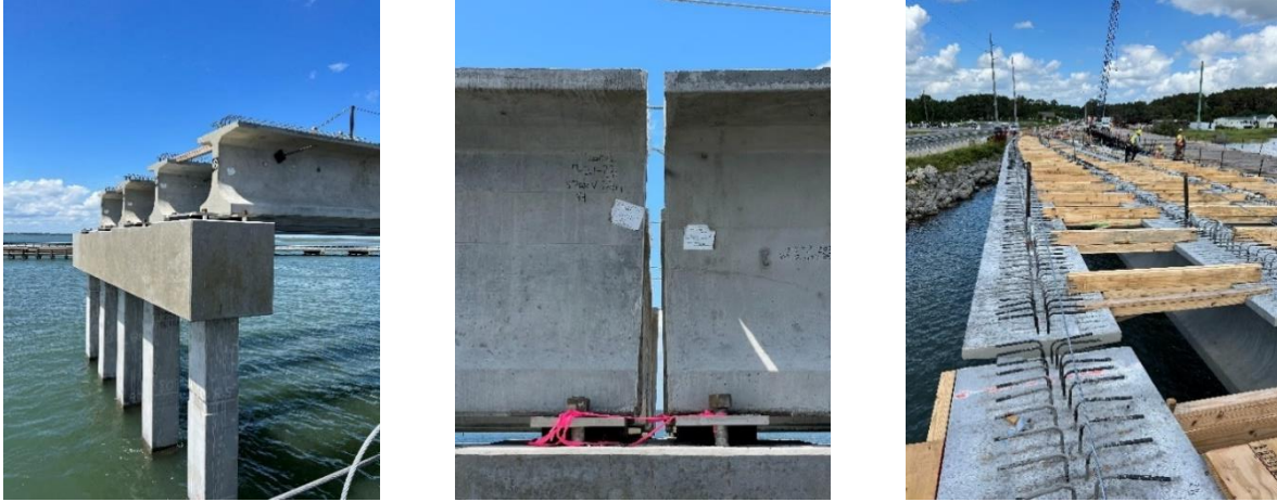
Figure A - 45. Girders in place
