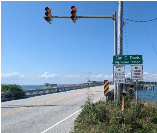
(a) Traffic interrupted by the swing-span
