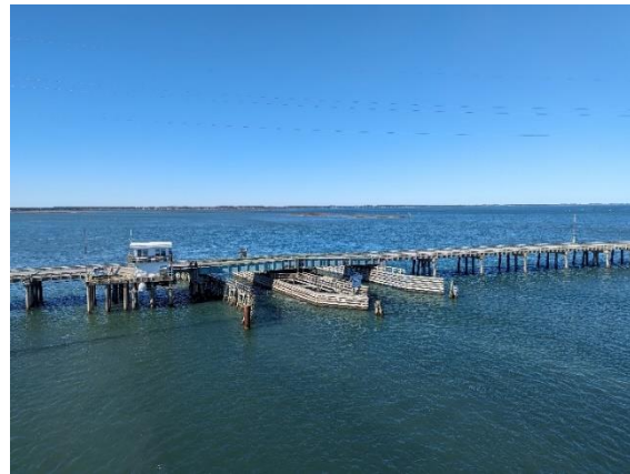
(b) Swing-span on Bridge No. 73
