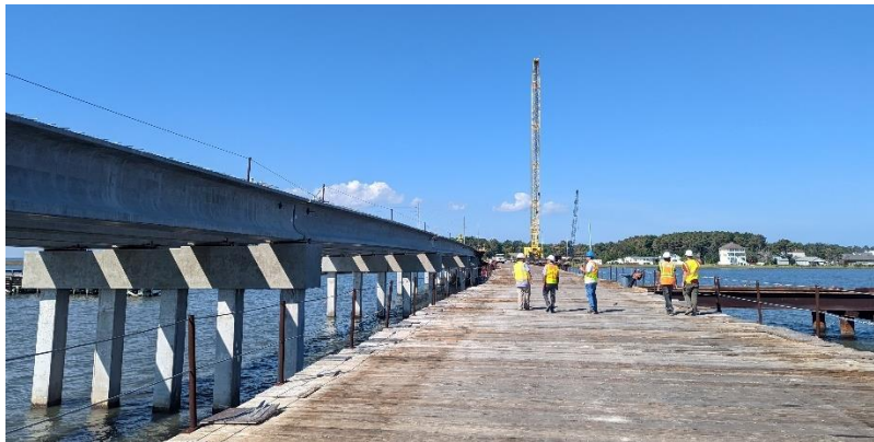
(c) Trestle parallel to the new alignment
