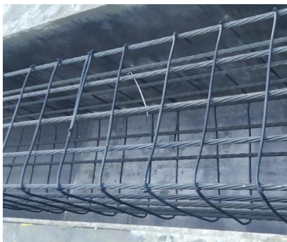
(a) CFRP spirals before casting
