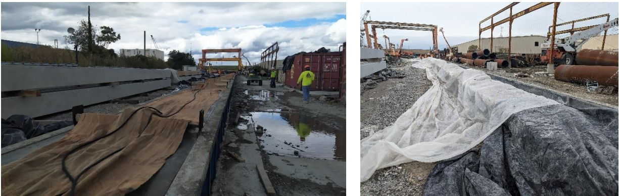
Figure A - 27. Concrete curing with thermal blankets
