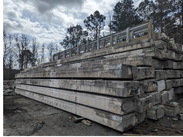
Figure A - 52. Demolished cored slabs from Bridge No. 73
