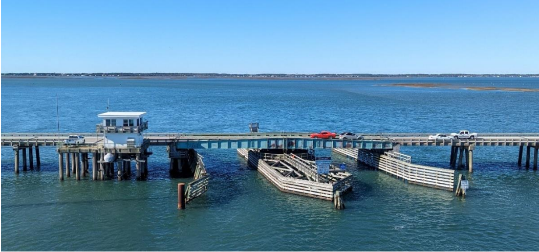
(a) Bridge No. 73 (Earl C. Davis Memorial Bridge) – Demolished
