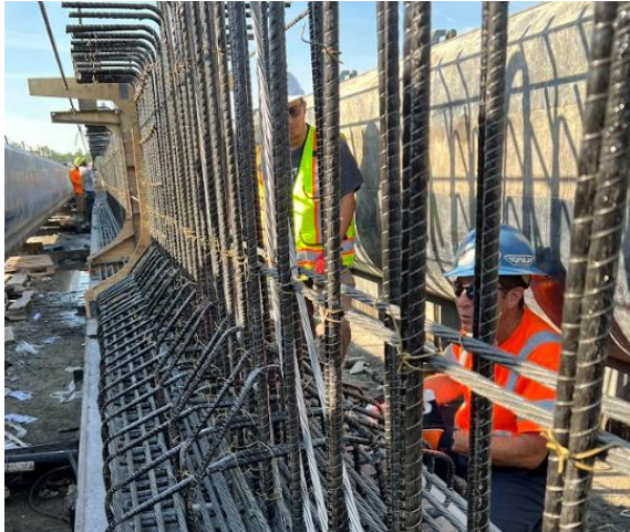
(a) FIB girders
