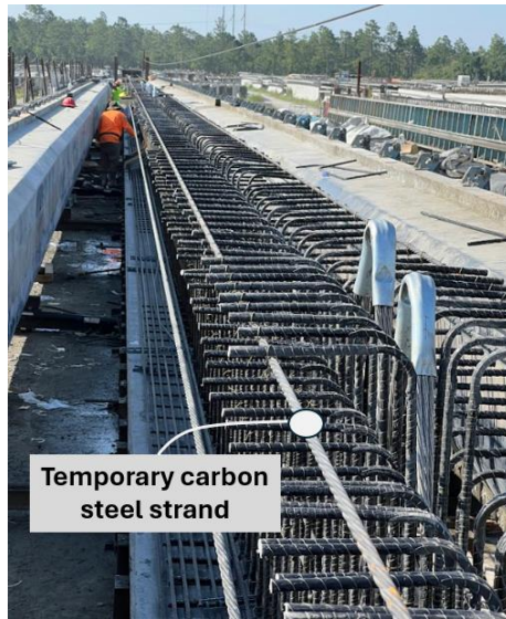
(a) Temporary steel strands
