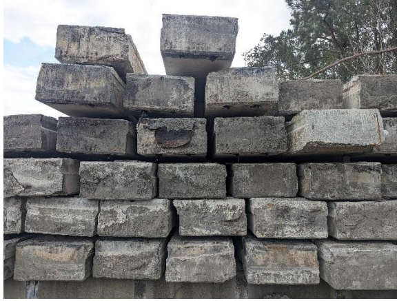
Figure A - 52. Demolished cored slabs from Bridge No. 73
