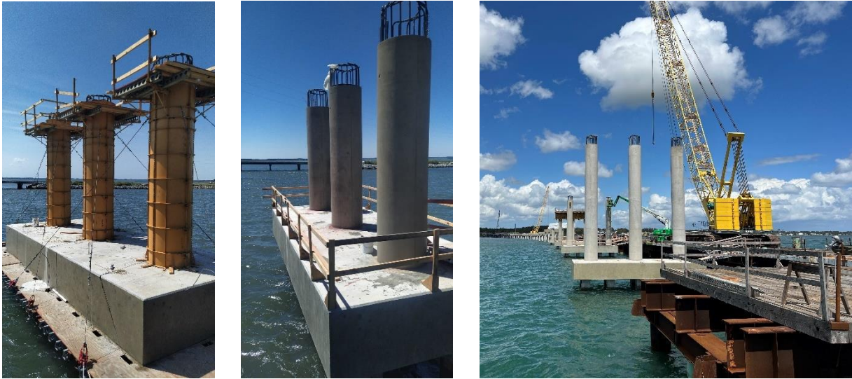
Figure A - 40. Pier columns
